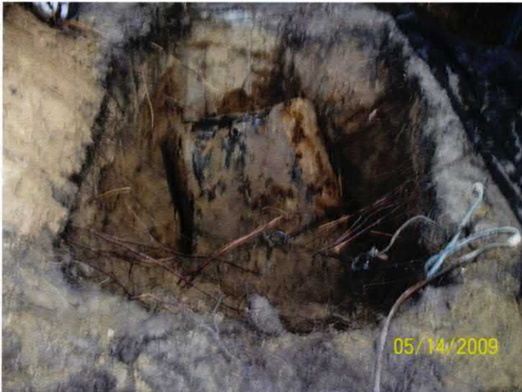
Picture 2: UST 1017Foxglove during removal from the excavation.
